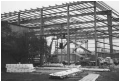
CONSTRUCTION OF NEW WAREHOUSE EXPANSION.
